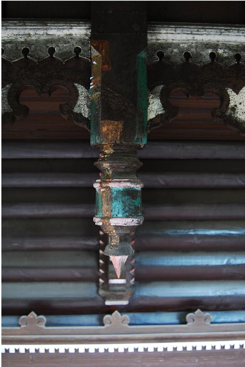
Abb.; 70 Foto Duras; September 2016; Fassade West, Fassungsbefund Zapfen
